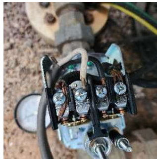
Water Treatment Equipment
